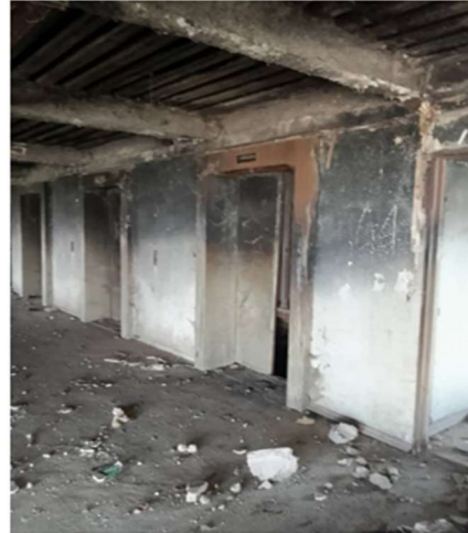
Plate 2: Hotel internal fire rated wall at lift area
