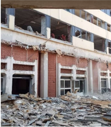
Plate 1: Hotel external wall constructed with Bricks and solid concrete block walls
