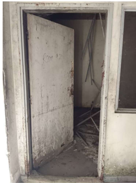
plate 6: Single door non fire rated door Source: Author's field work (2024)
