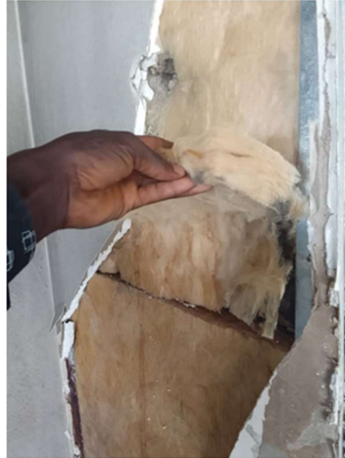
Plate 4: Hotel internal fire rated wall
