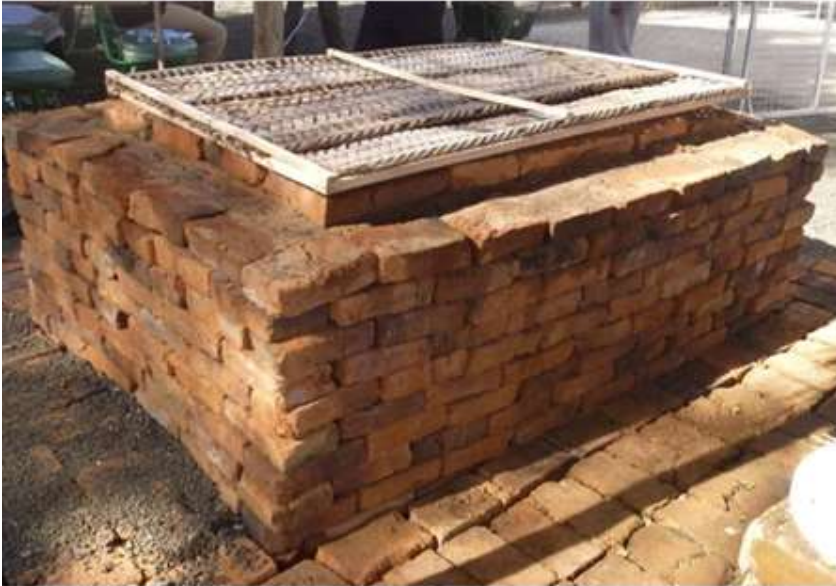
Fig.4: Zero-Energy Cooling Chamber for storage of fresh fruits and vegetables in Tanzania
