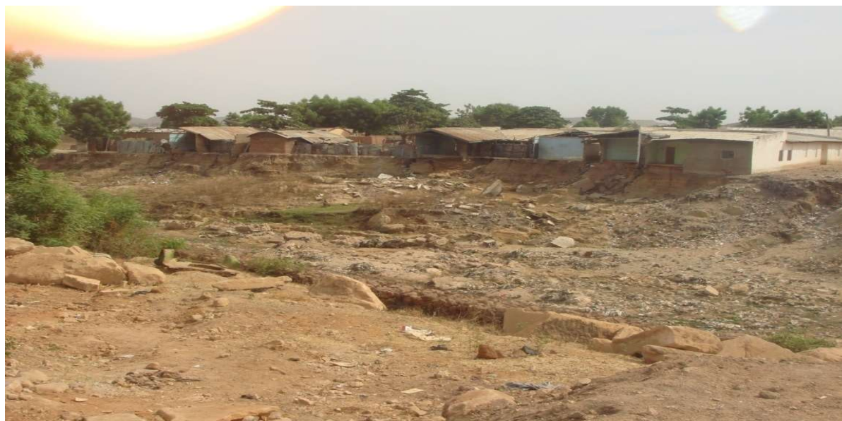
Plate 1: Gully threatening houses in Kumo
