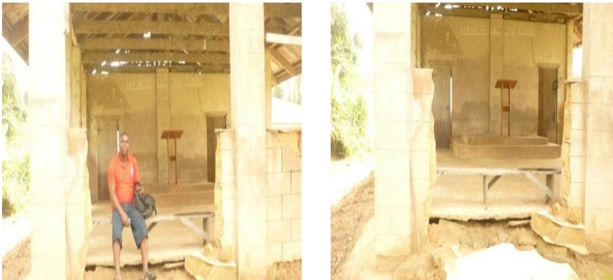
Fig.1: Odual Native Court Building
