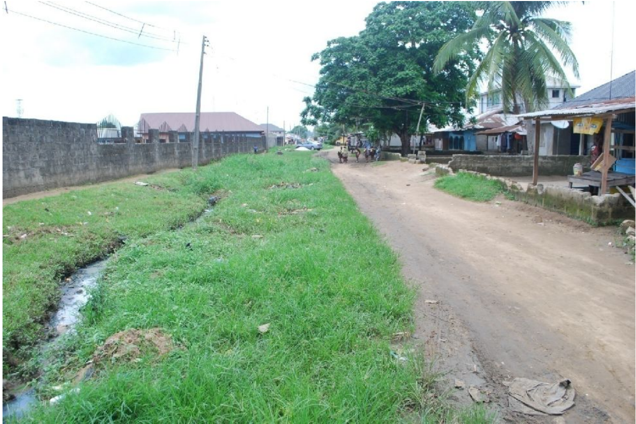
Fig. 5a: Ineffective Drainage on Gokana Street of the Study Area
