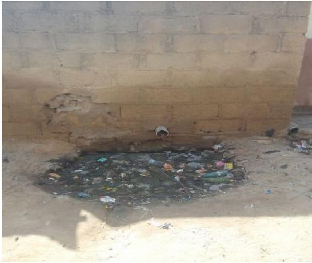
Plate 1: Cesspool for disposing grey water in water in Gaboru ward
